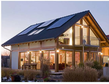
Off grid power system
